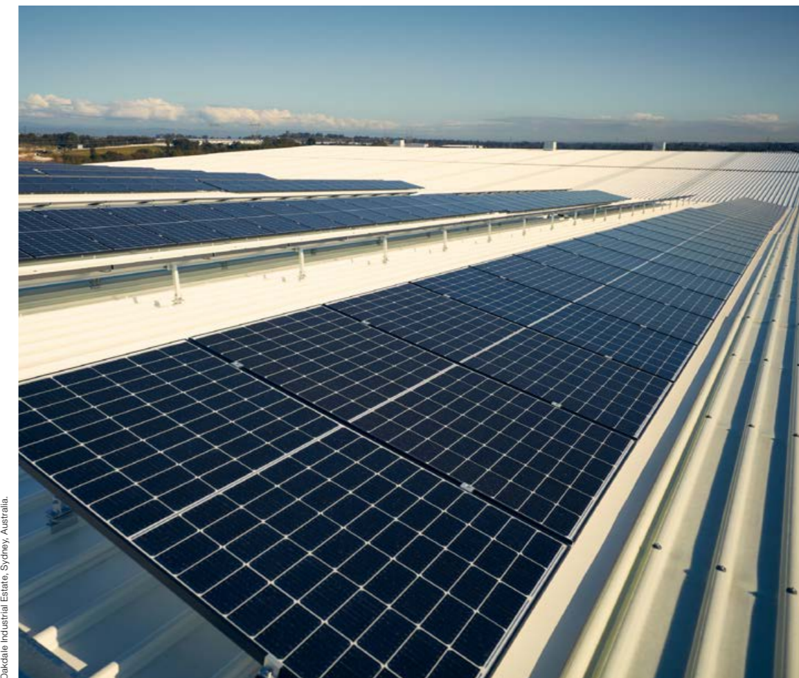
Oakdale Industrial Estate, Sydney, Australia.
