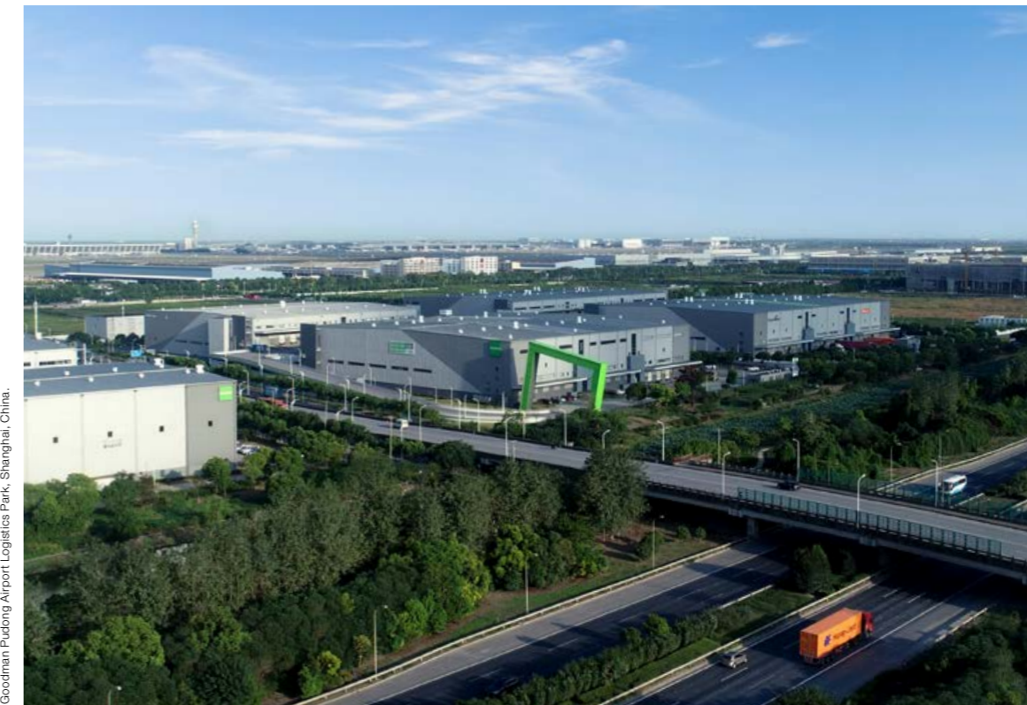
Goodman Pudong Airport Logistics Park, Shanghai, China.
