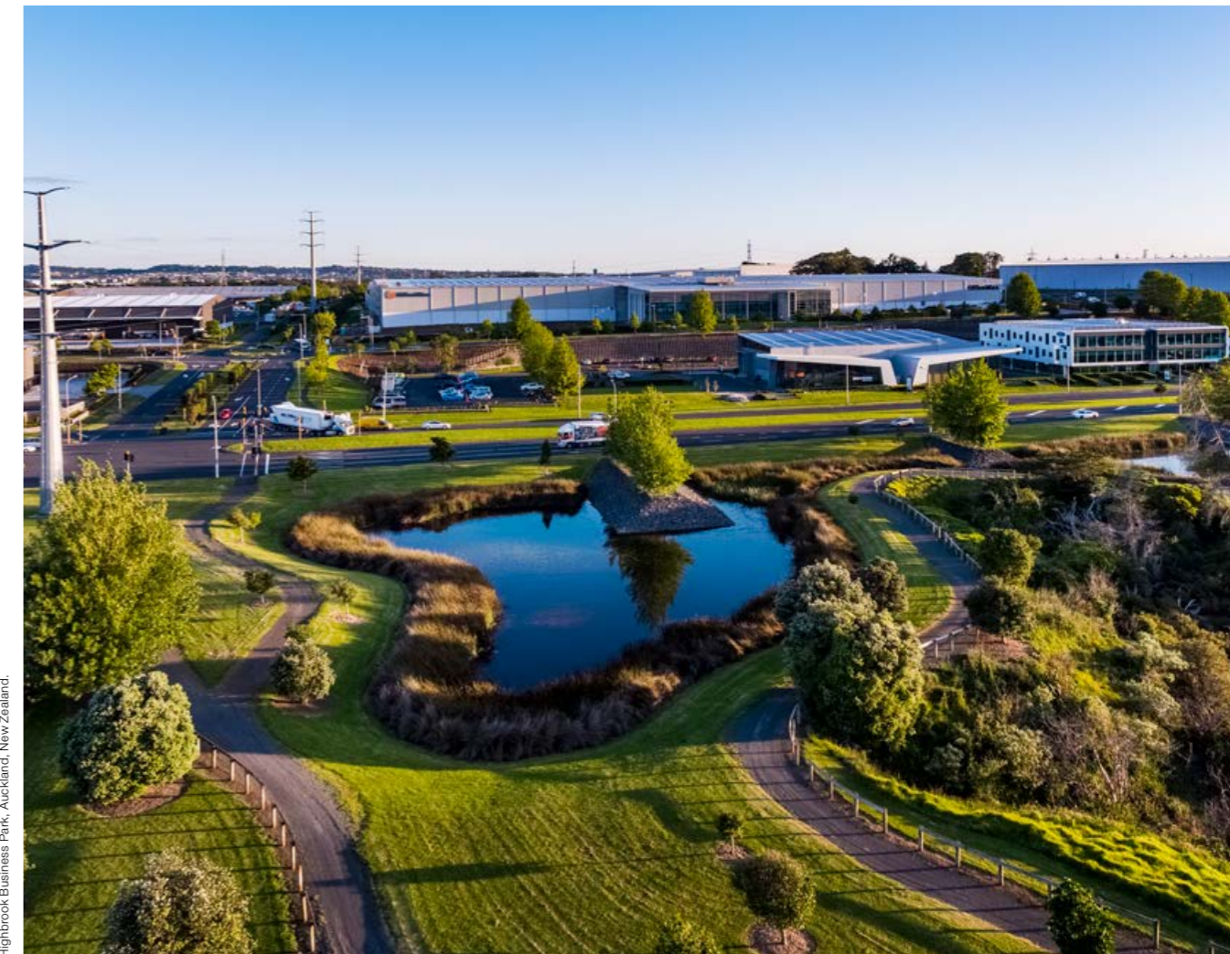
Highbrook Business Park, Auckland, New Zealand.
