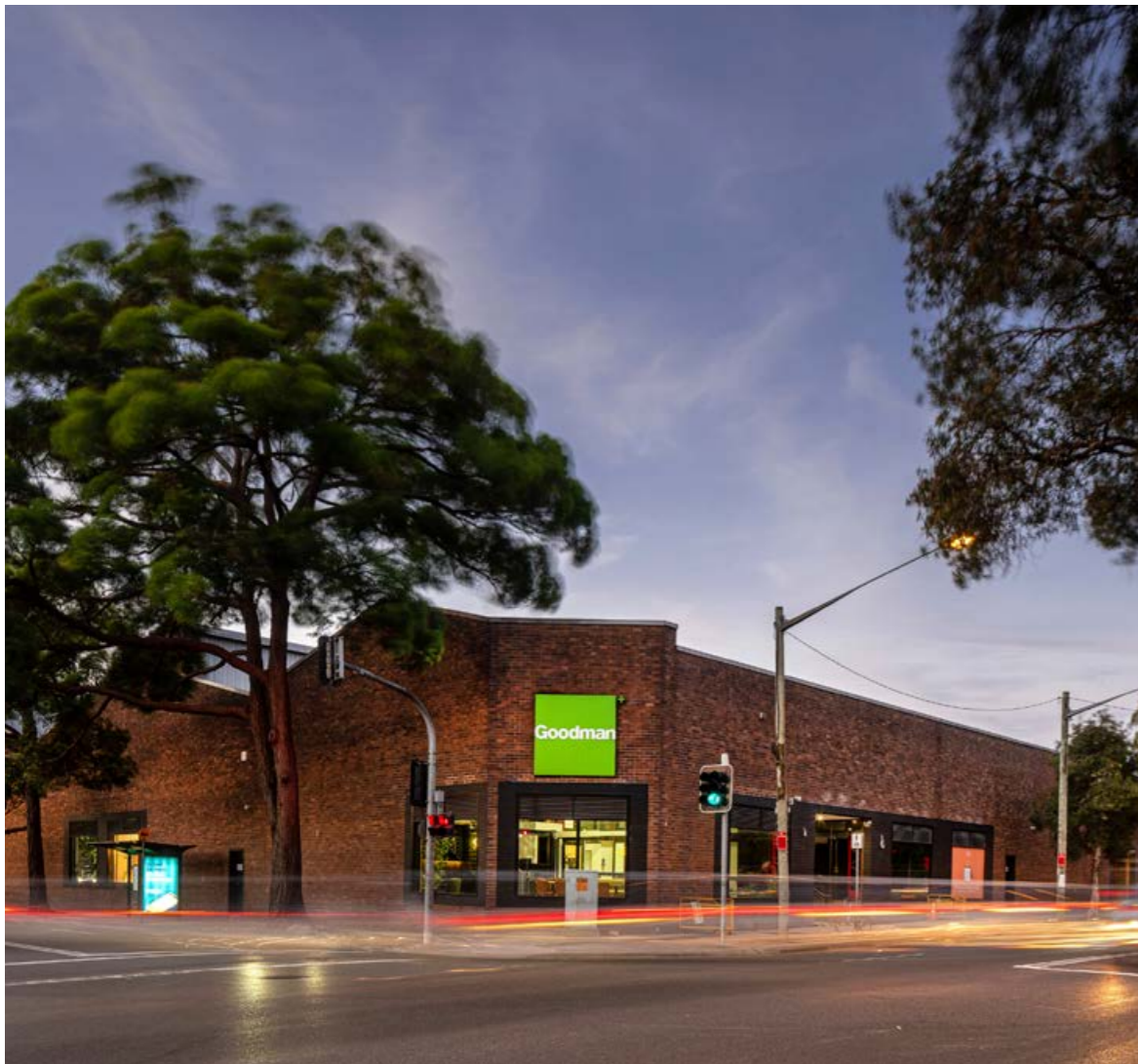
Alexandria Industrial Estate, Sydney, Australia.
