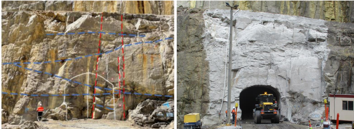
Figure 17: Mapping of the dominant geotechnical features in the exploration decline portal face (left) and the established exploration decline portal (right)
