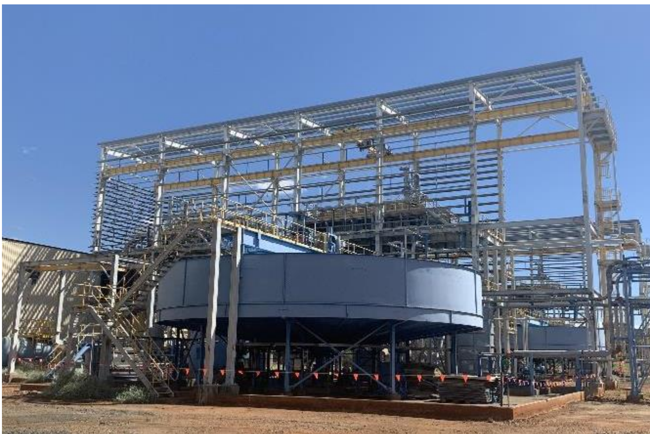
Figure 5: Tailings Filtration system including filter press (background) and thickener (foreground) that PNX is assessing for use at the Fountain Head project. The equipment would be transported and reconstructed at Fountain Head.
