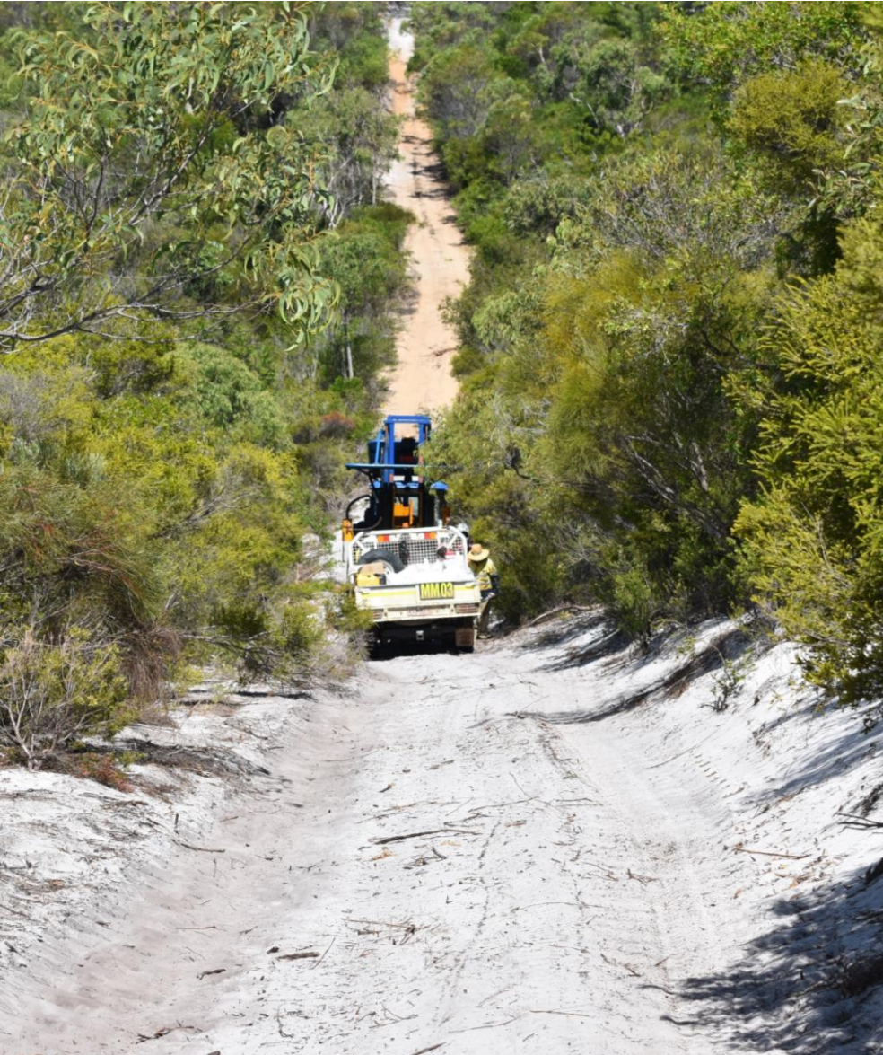
Figure 3: photo of Yearlong Contractors vacuum-based drill rig working at CFS project
