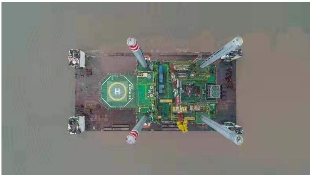
Aerial view of platform HYSY 163 mounted on dry tow barge
