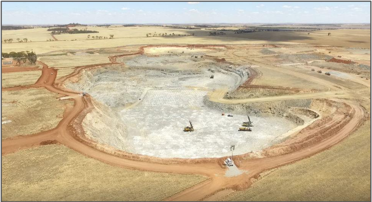
Figure 4: Tampia Pit looking South
