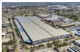
$200.2m 56-88 LISBON STREET, FAIRFIELD, NSW DISTRIBUTION CENTRE
