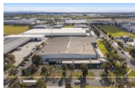
$20.6m 30 FULTON DRIVE, DERRIMUT, VIC DISTRIBUTION CENTRE
