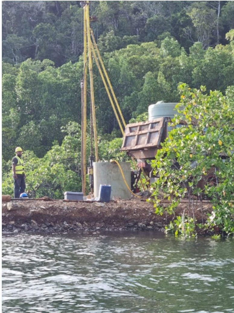
Photo 5. Geotechnical drilling for wharf construction
