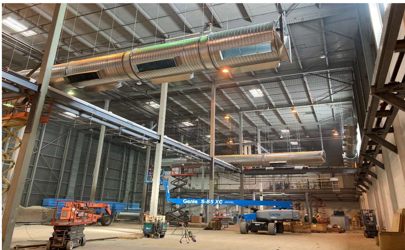
Figure 3: High Bay Mechanical Utilities Ductwork Installation
