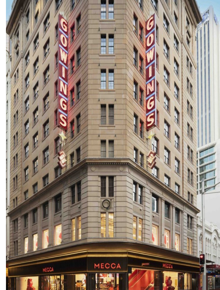
THE GOWINGS BUILDING
