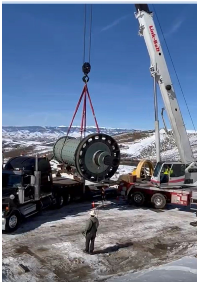
Figure 7: The 250tpd ball mill being unloaded at the Lucky Strike site in Colorado
