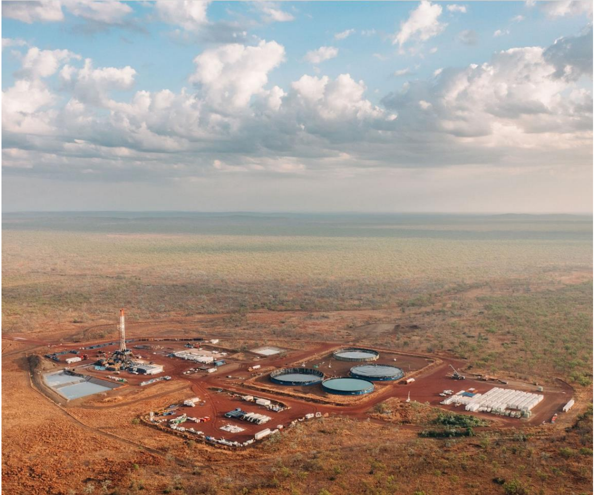
Figure 1: Drilling operations completing in EP 161, November 2021
