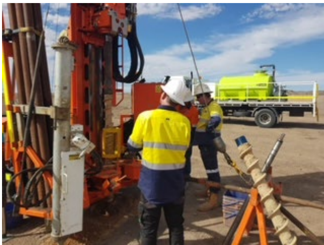
Drill rigs and teams geotechnical investigations associated with the construction of the Leigh Creek Urea Project (LCUP) gasification wells and power generator areas.
