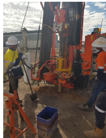
Drill rigs and teams geotechnical investigations associated with the construction of the Leigh Creek Urea Project (LCUP) gasification wells and power generator areas.
