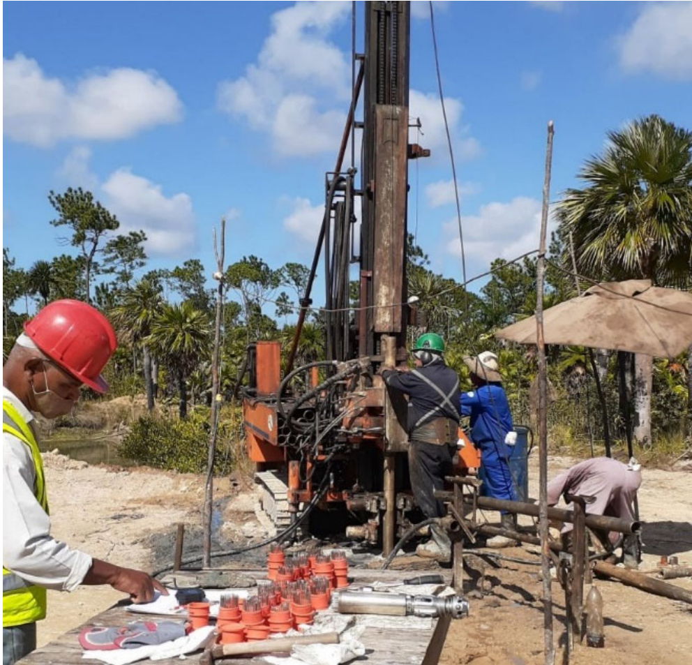
Drilling at La Demajagua
