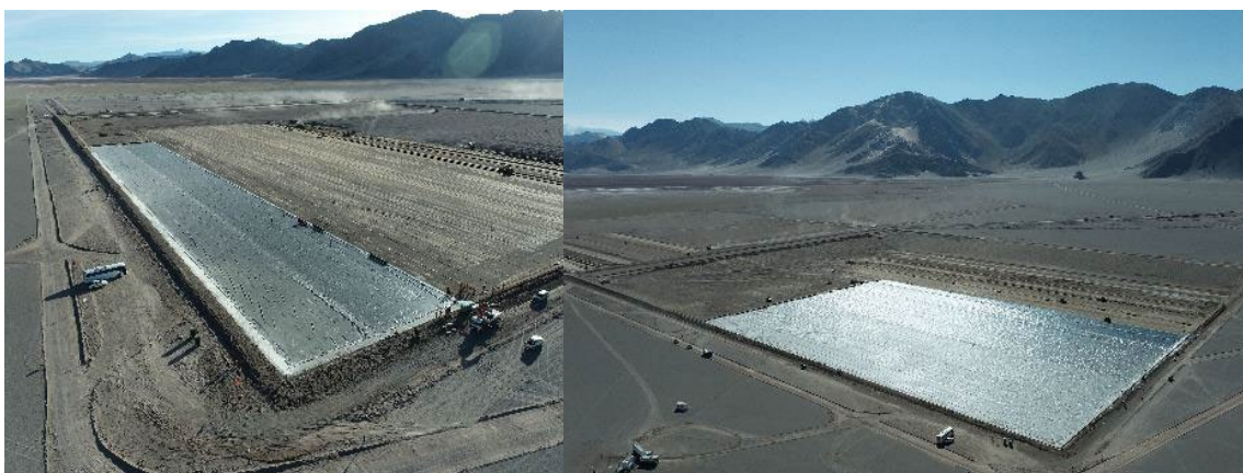
Figure 2: Sal de Vida – pond construction underway
