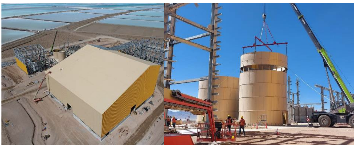
Figure 1: Olaroz Stage 2 - construction 77% complete
