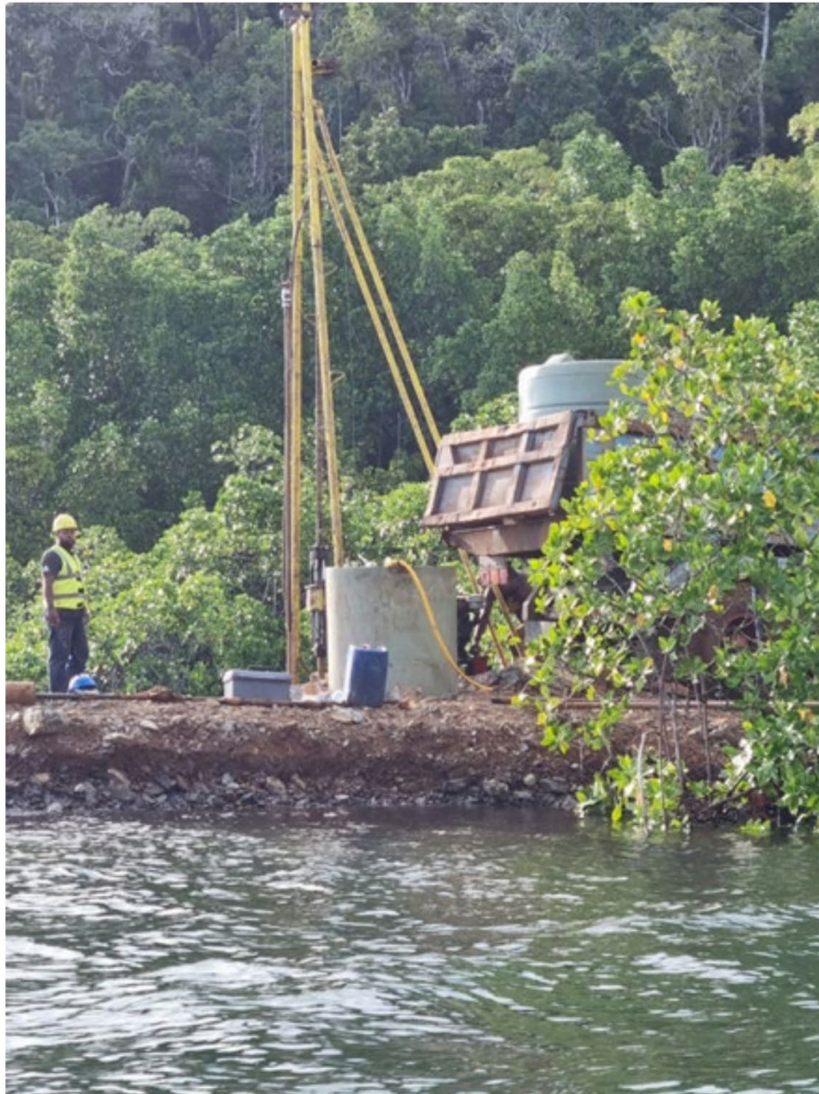
Photo 5. Geotechnical Drilling for Wharf Construction
