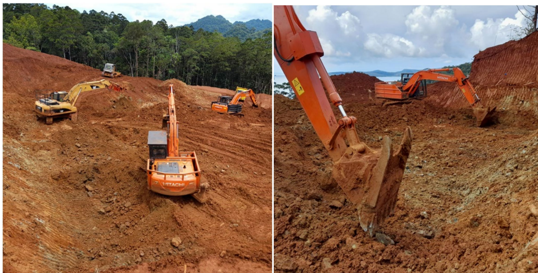
Photo 2. Mining of Test Pits
