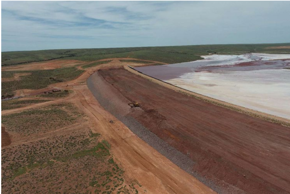
Figure 15: TSF Stage 2 embankment progress
