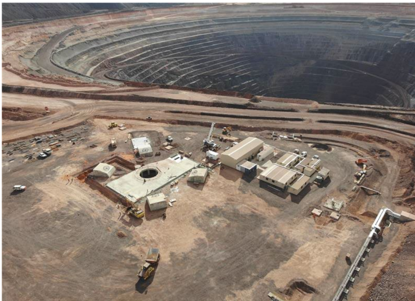
Figure 9: Shaft collar construction site works complete
