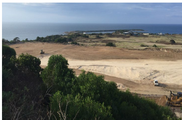
Process plant earthworks nearing completion: March 22
