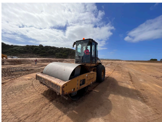
Compaction rolling of process plant area: Mar 22
