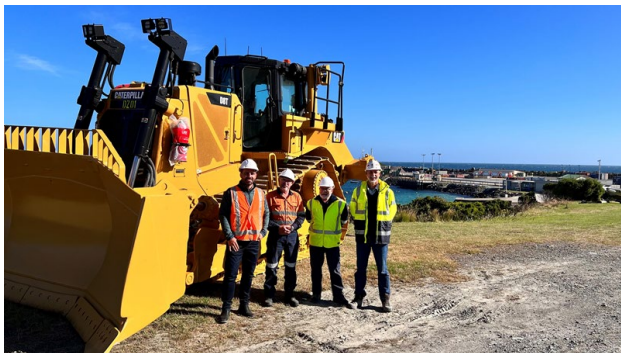
DZ01 Dozer arriving on site to start earthworks: Jan 22
