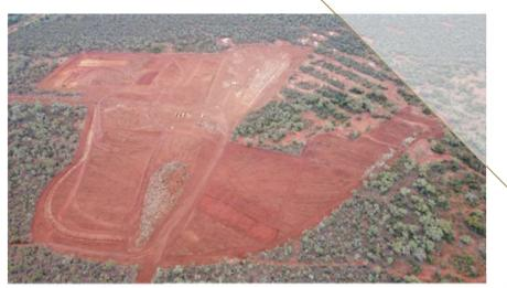
Neill Earthmoving cleared and grubbed 32 hectares of land, established access roads, and commenced excavation for the box cut.
