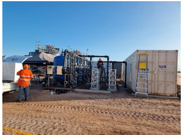
Figure 1 – Installation of reverse osmosis plant
