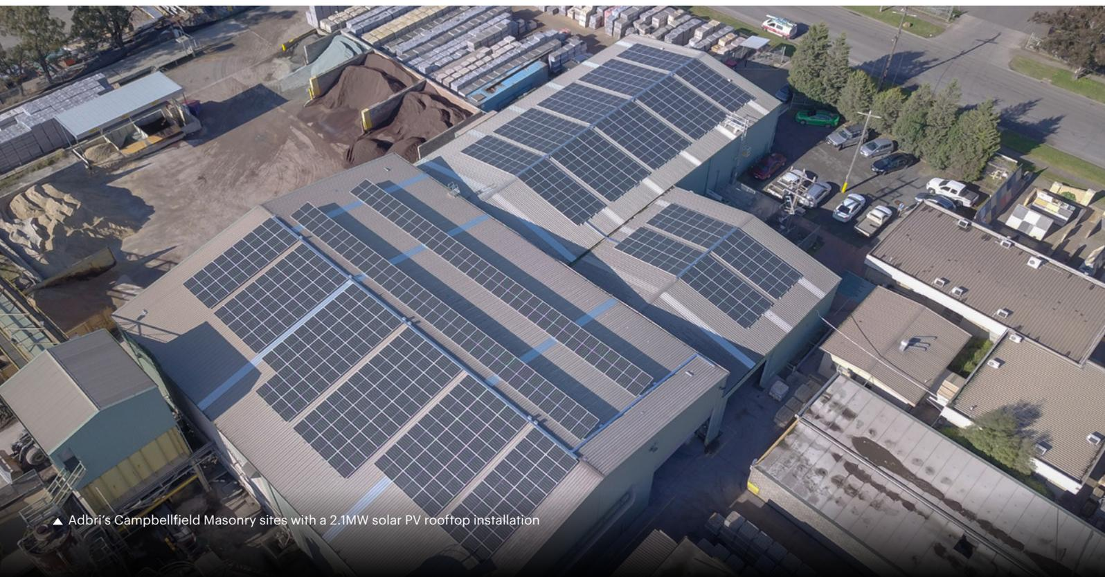
▲ Adbri's Campbellfield Masonry sites with a 2.1MW solar PV rooftop installation
