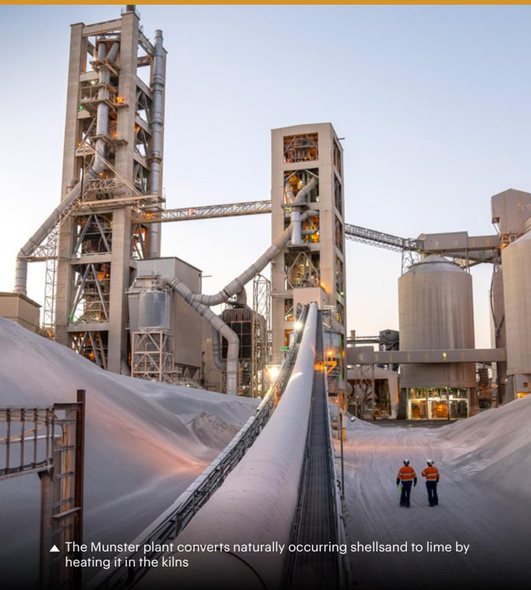
▲ The Munster plant converts naturally occurring shellsand to lime by heating it in the kilns
