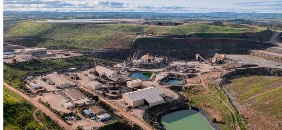
3.6MTPA PROCESSING PLANT
