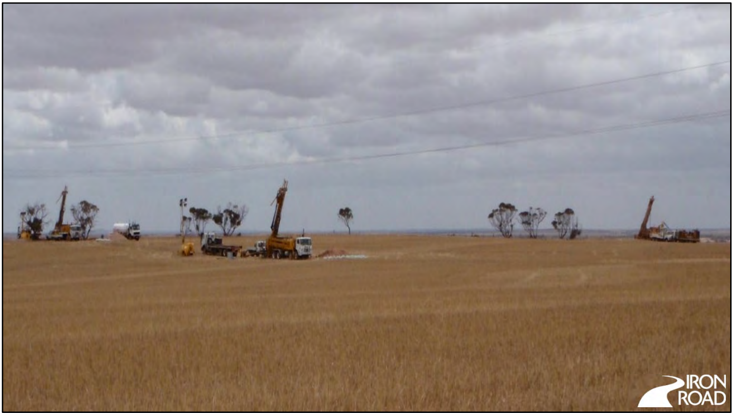
Diamond drills oriented at -60^{\circ} true north.
