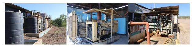
Figure 1. (a) Civil works will include repair of the existing bunds (b) side by side generators and (c) Generator and chiller compressor housing.
