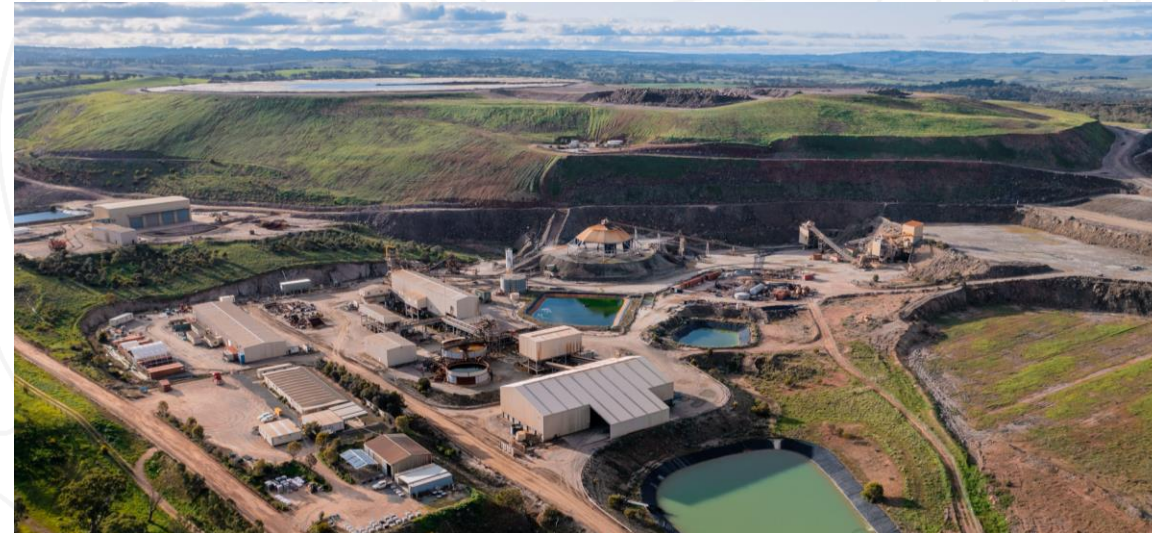
3.6MTPA PROCESSING PLANT
