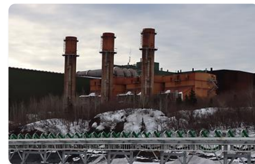
Pointe Noire Pelletizing Facility
