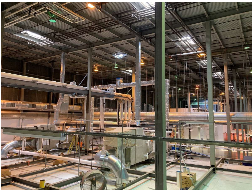
Figure 3: Air Handling Unit (AHU) ductwork installation
