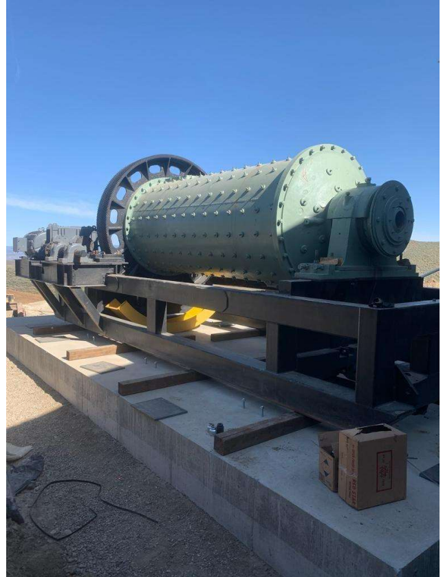
Figure 3: Ball mill placed in final position on concrete pad
