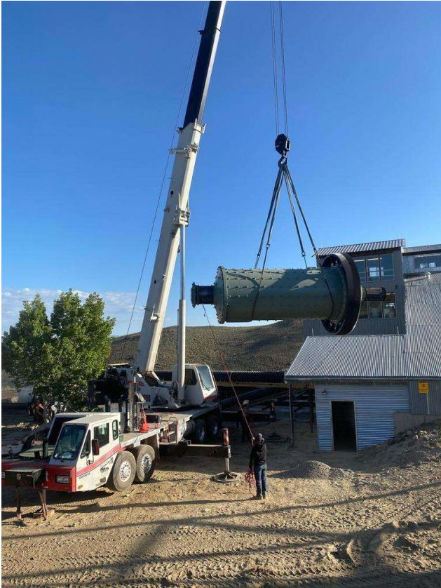
Figure 2: 250 tonne per day ball mill being craned
