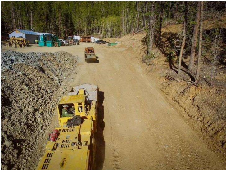
Figure 4: Material from the Gold Links being stockpiled
