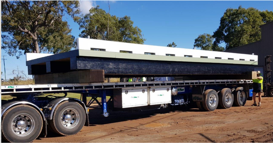
Bridge Systems 170mm thick Plywood Deck & 600mm thick LVL beams
