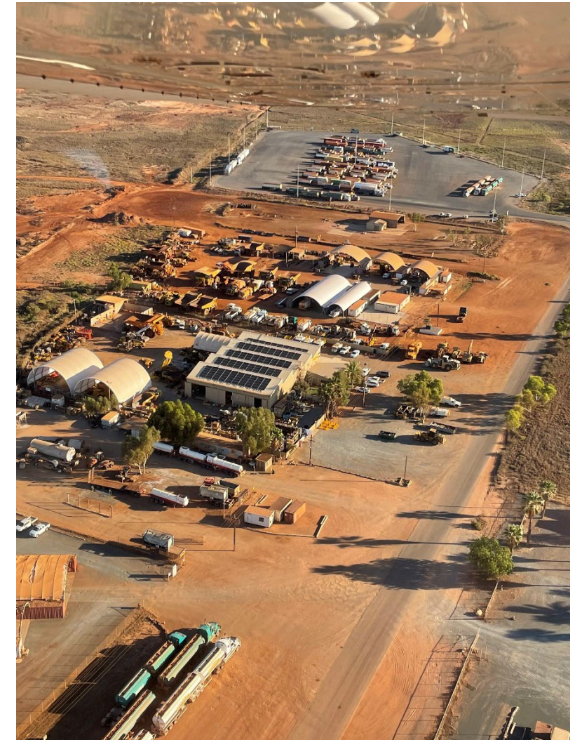
WesTrac 150kW solar array at Port Hedland
