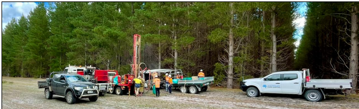
Figure 2 – RC/air-core drilling in progress on site
