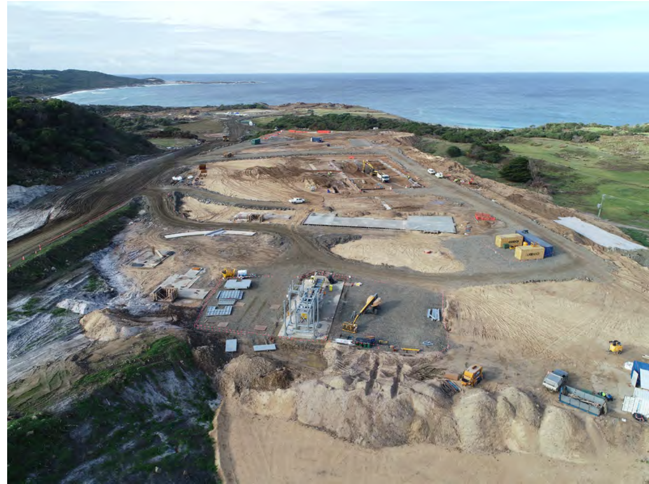
Status of Process Plant Construction July 2022
