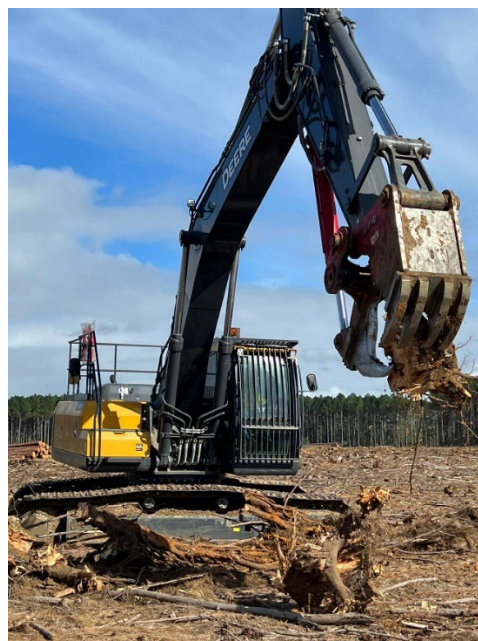
New stump pulling equipment, the “T-rex”
