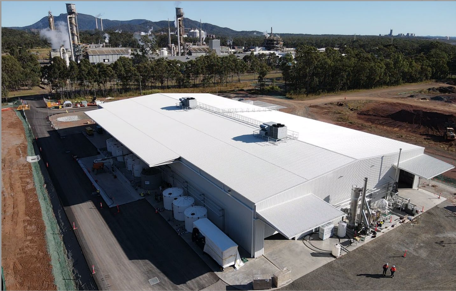
Stage 1 PPF building – July 2022
