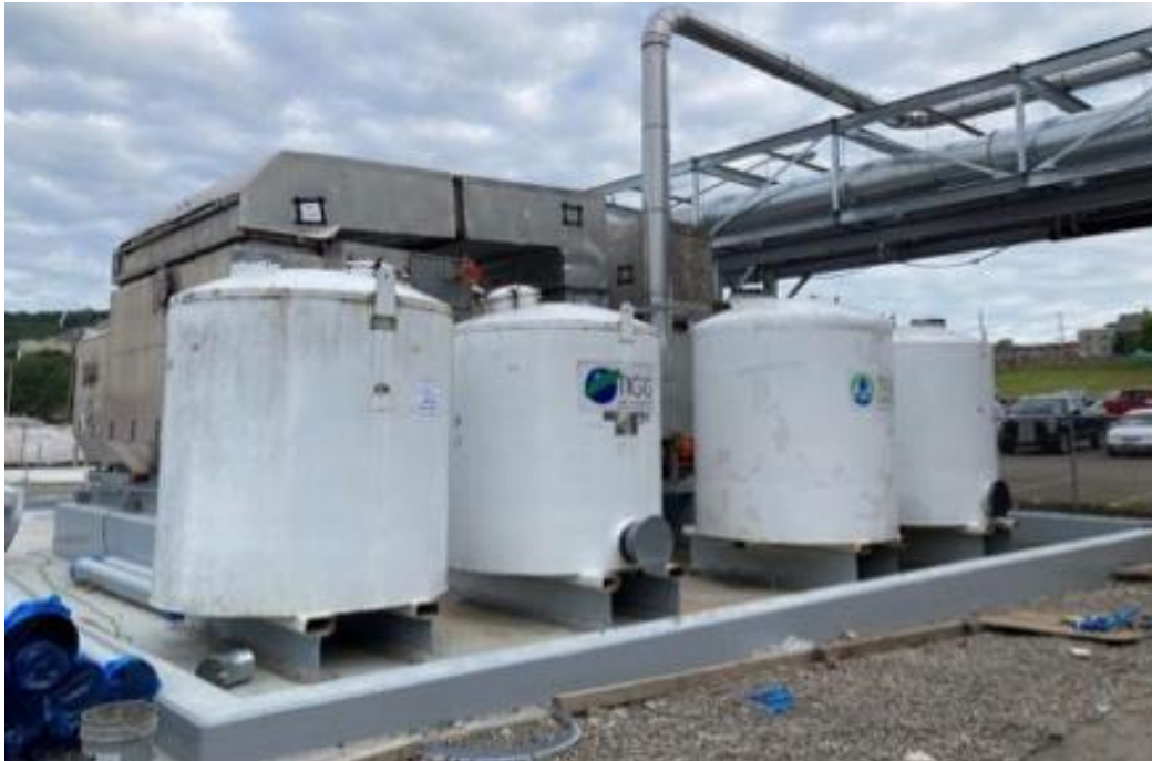
Figure 3: Condenser system with carbon to capture solvent
