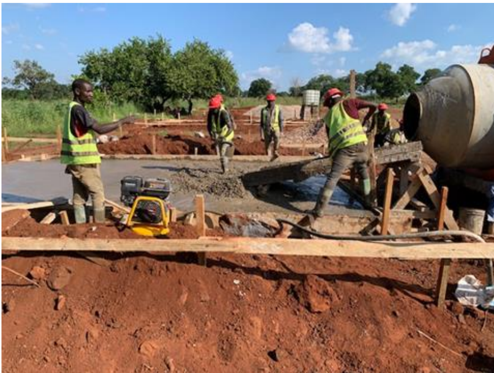
Figure 5: Concreting Works on site
