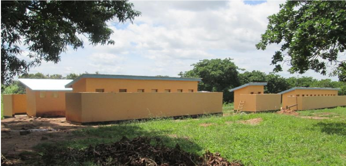
Figure 7: Matambarale Primary School Toilet Block
