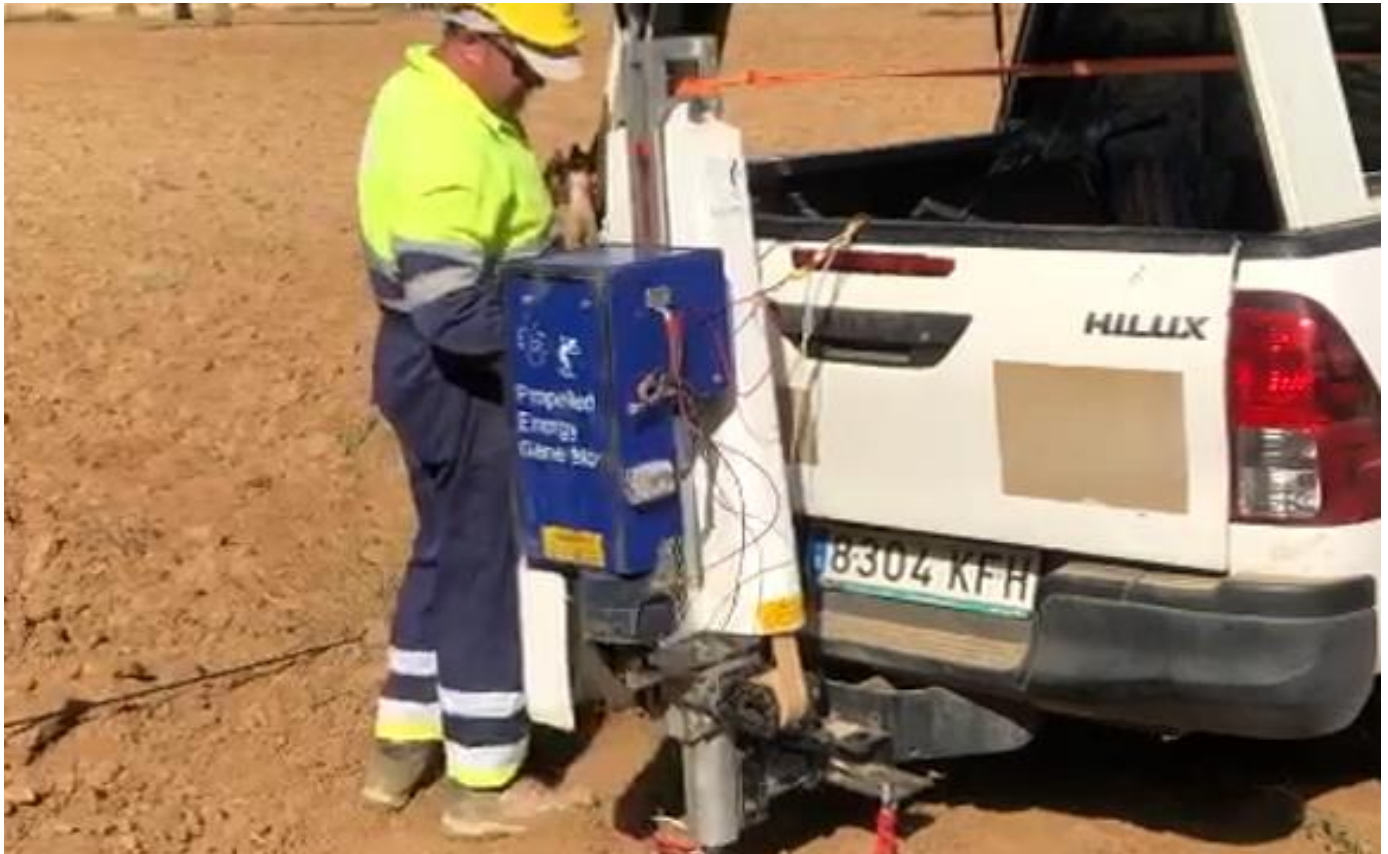
Figure 3. Seismic investigations on process plant pad
