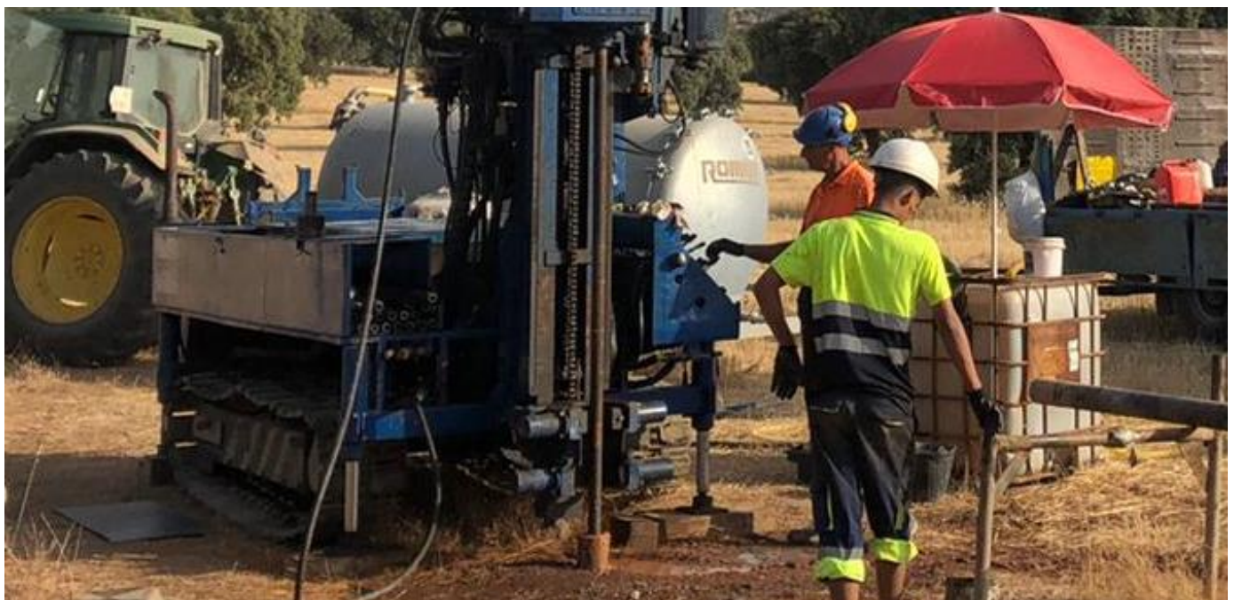
Figure 1. Civil Investigations (GT Rig) Tailings Dam footings
