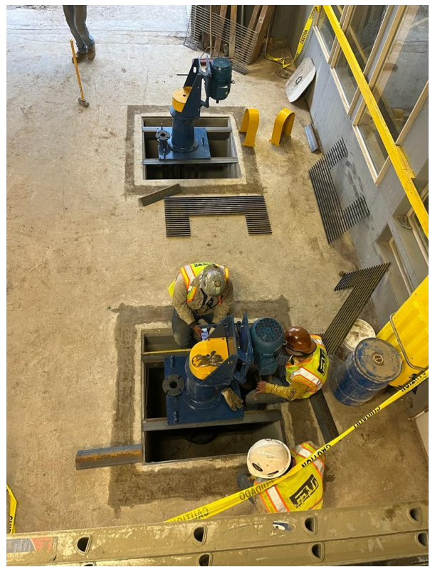
Figure 8b: Upgraded pumps being installed
