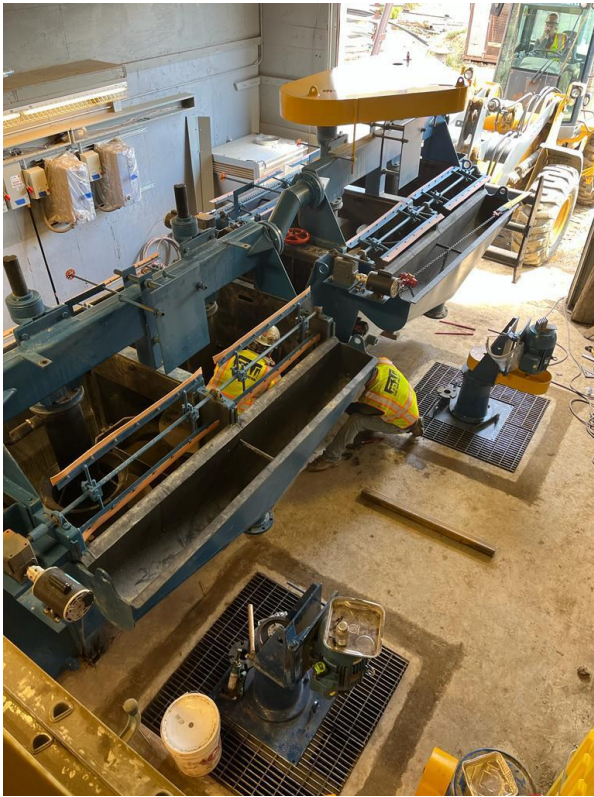
Figure 8a: Upgraded flotation cells being installed
