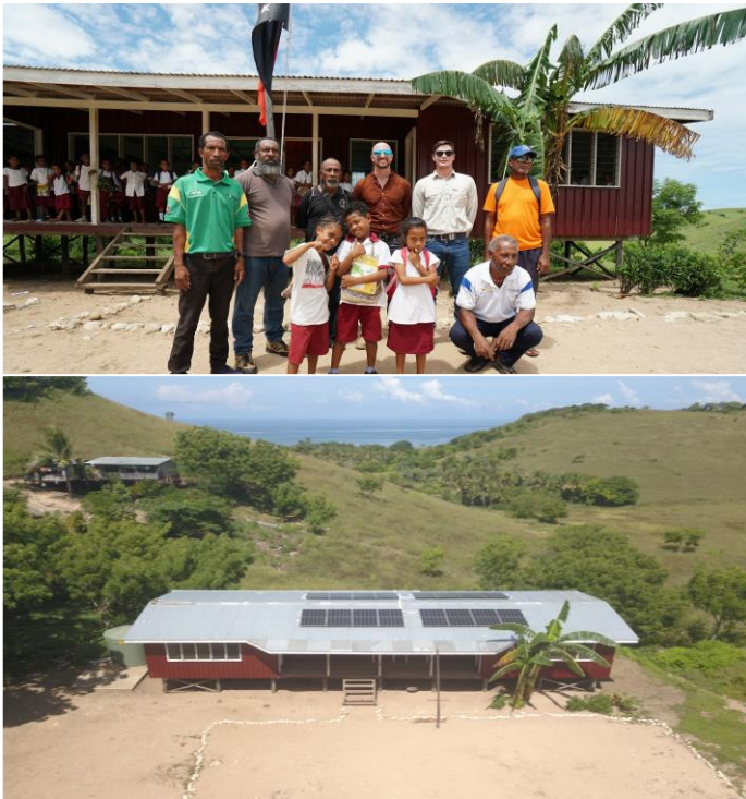
Mayur team with local community after installation of first ever microgrid solar at Kido school
