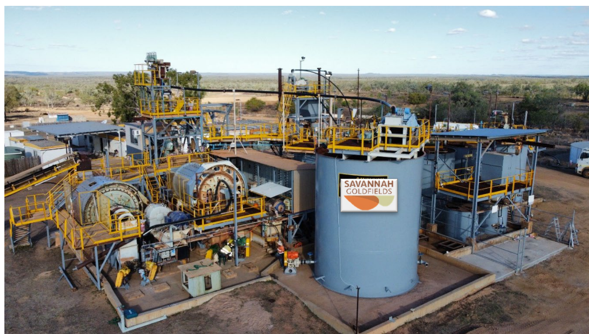
Georgetown Gold Processing Plant
