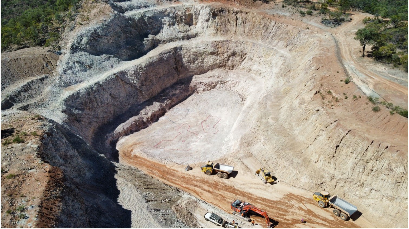
Open cut pit at Agate Creek
