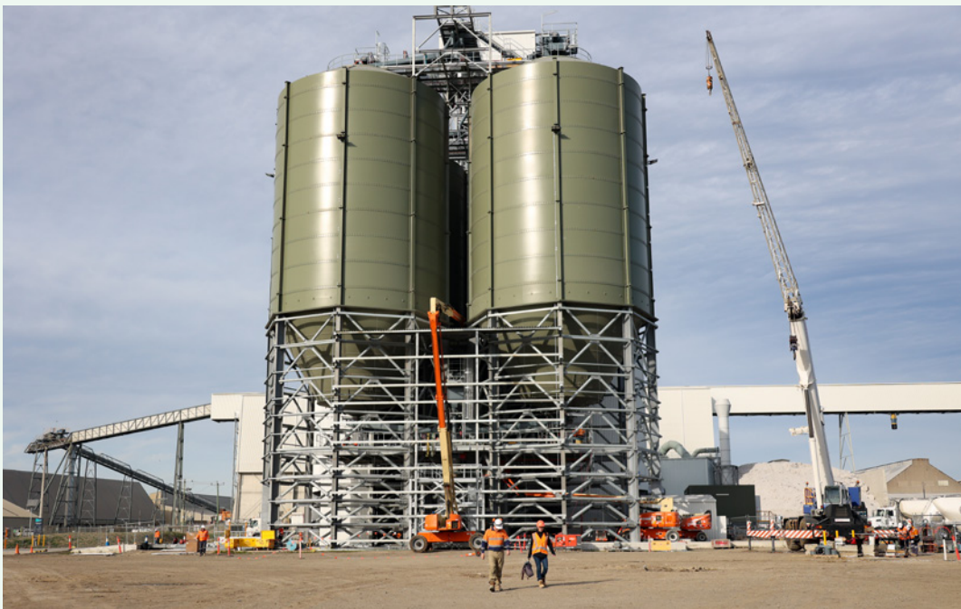
Geelong Cement grinding and storage facility, Vic
