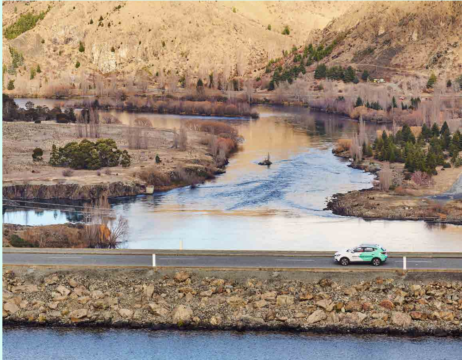
Benmore Hydro Power Station, Otematata.
