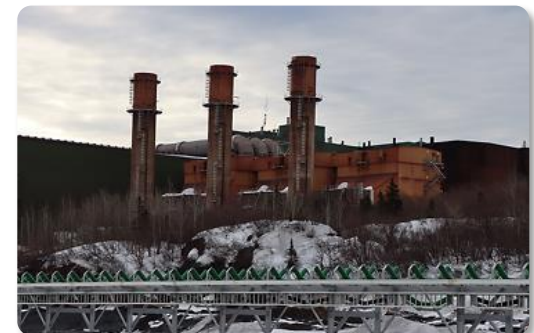
Pointe Noire Pelletizing Facility
