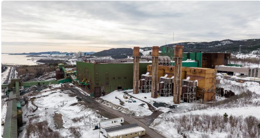
Pointe Noire Pelletizing Facility
