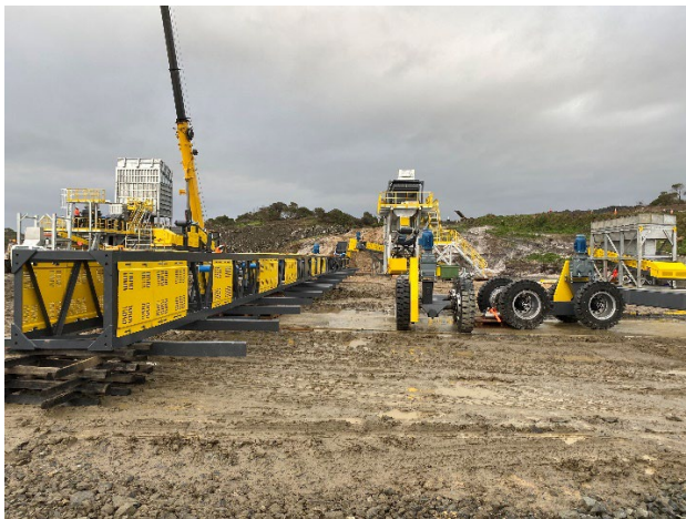
Figure 4 - Installation of Fine Ore Slewing Conveyor
