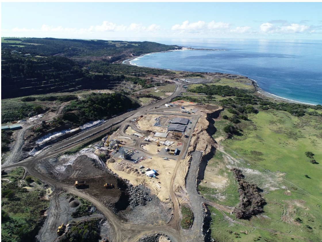
Figure 1 - Aerial Photo of Process Plant Area (Looking North-East)
