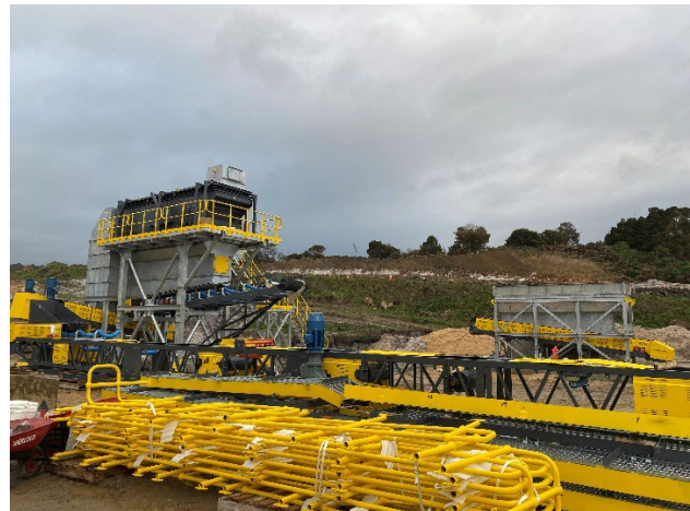
Figure 3 - Installation of Secondary Screen
