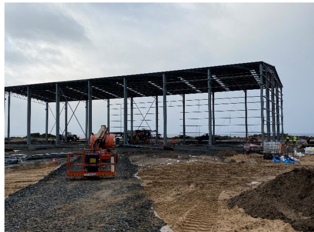
Figure 5 - Erection of Main Process Building
