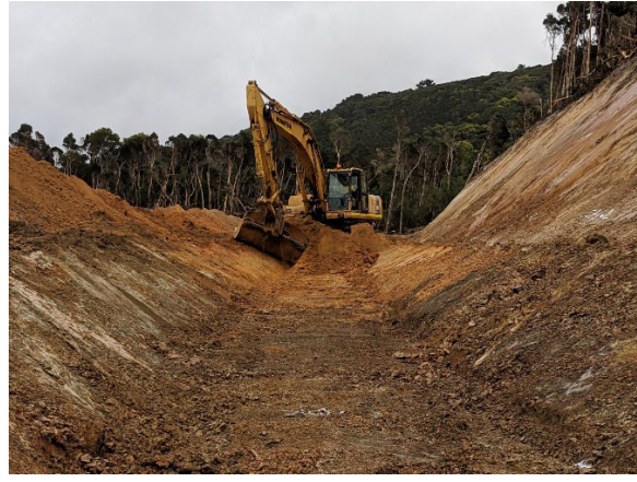
Figure 7 - Earthworks for Tailings Storage Facility
