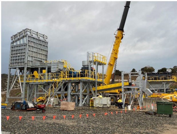
Figure 2 - Installation of Primary and Secondary Crushing Equipment
