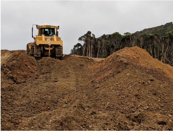
Figure 6 - Earthworks for Tailings Storage Facility
