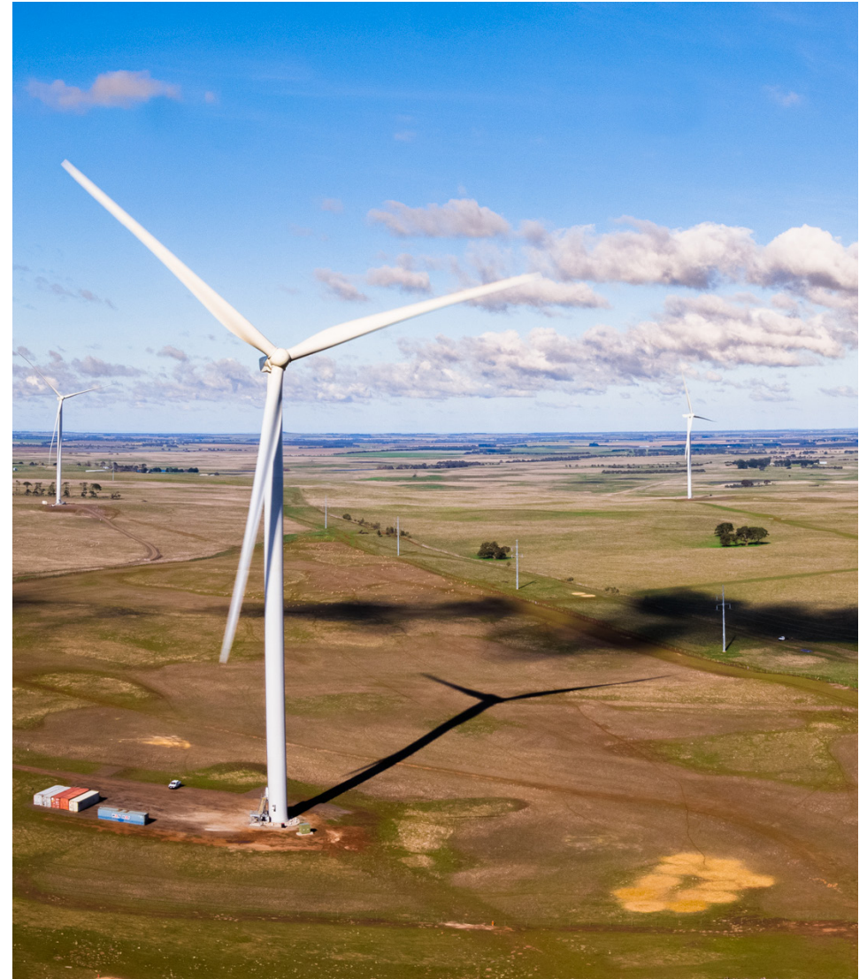
Stockyard Hill Wind Farm
