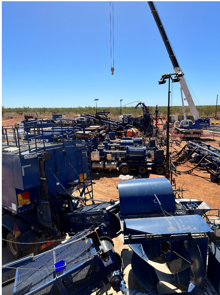
Schlumberger hydraulic fracturing spread at Carpentaria-2H well pad
