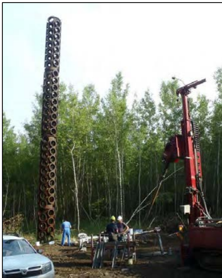
Figure 6-4: Historical Decantation Tower Located on Cell #3, Near Drill Holes T3-310, 311, and-318
