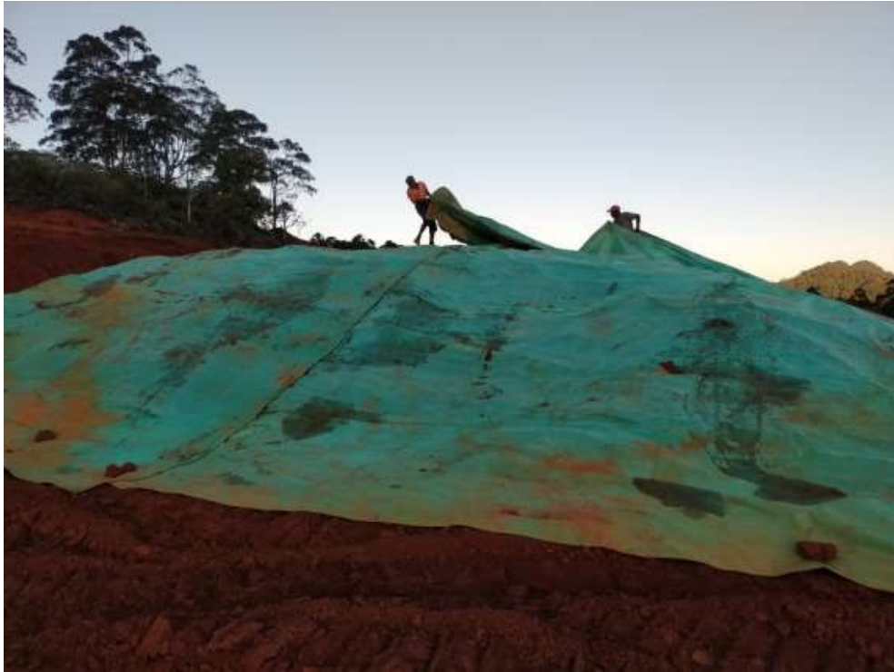
Photo: Tarpaulins placed over completed stockpile
