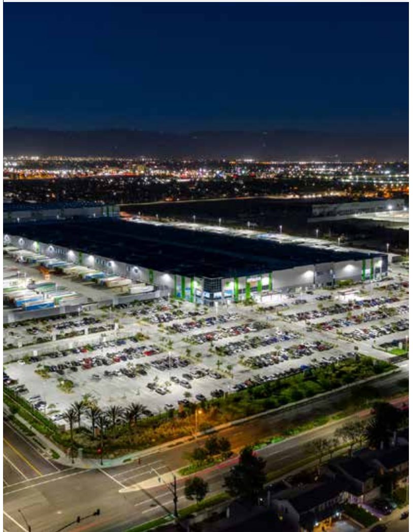
Goodman Logistics Center Fontana II, Los Angeles, USA.
