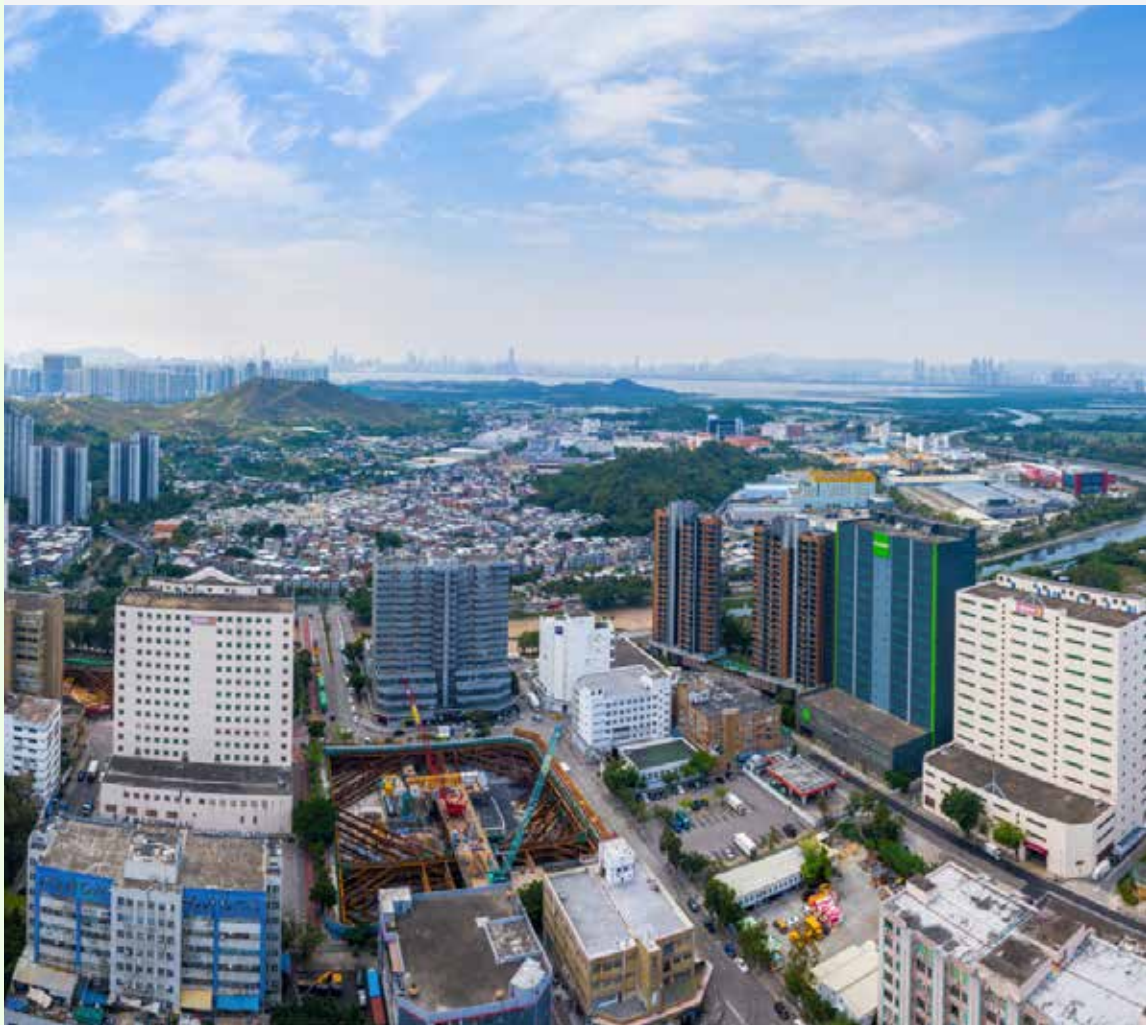
Goodman Yuen Long Logistics Centre, Hong Kong SAR, China.
