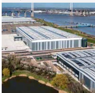
Crossways Commercial Park, Greater London, UK.
