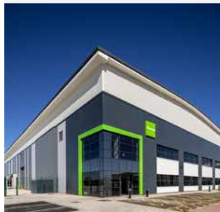
Crossways Commercial Park, Greater London, UK.
