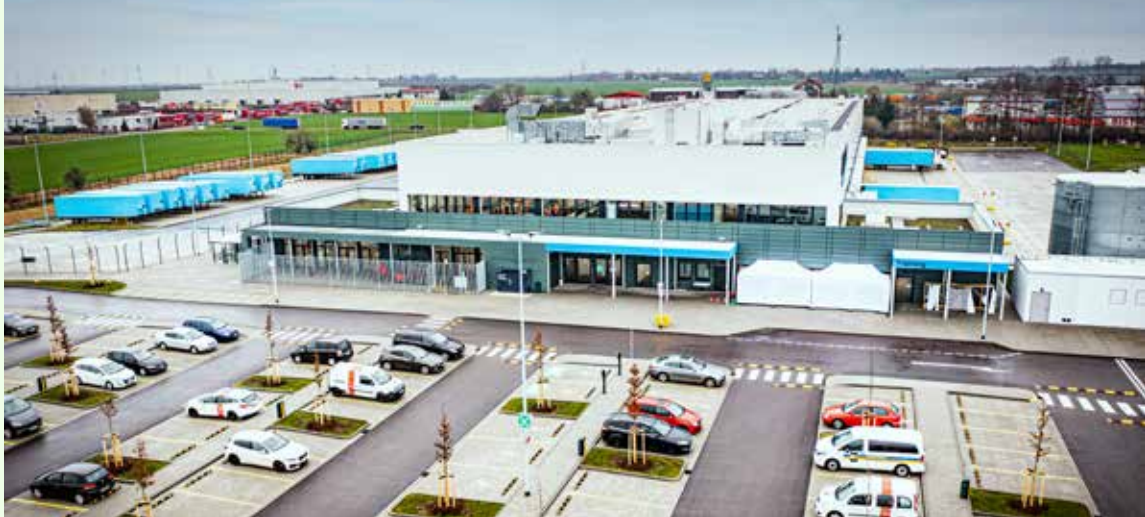
Halle VI Logistics Centre, Halle, Germany.
