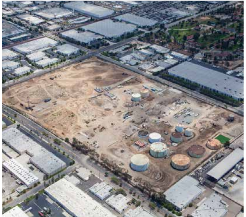
(Before) Goodman Commerce Center Santa Fe Springs, Los Angeles, USA.
