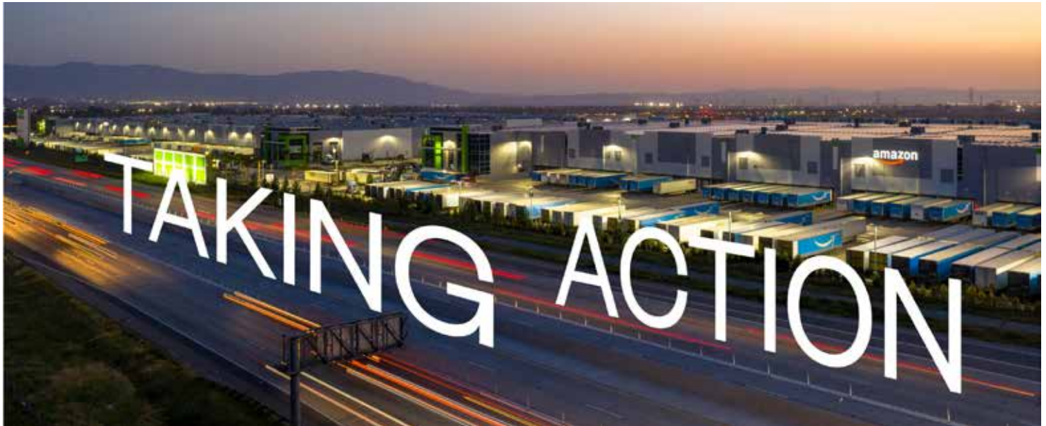
Goodman Commerce Center Eastvale, Los Angeles, USA.
