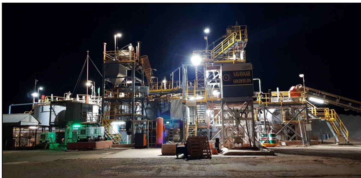
Georgetown Gold Processing Plant
