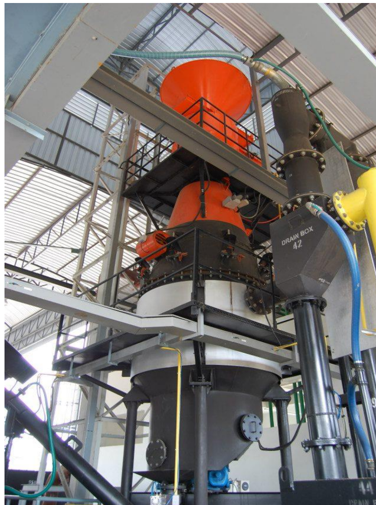
A Patriot EPC Contractor Gasifier type under going installation
